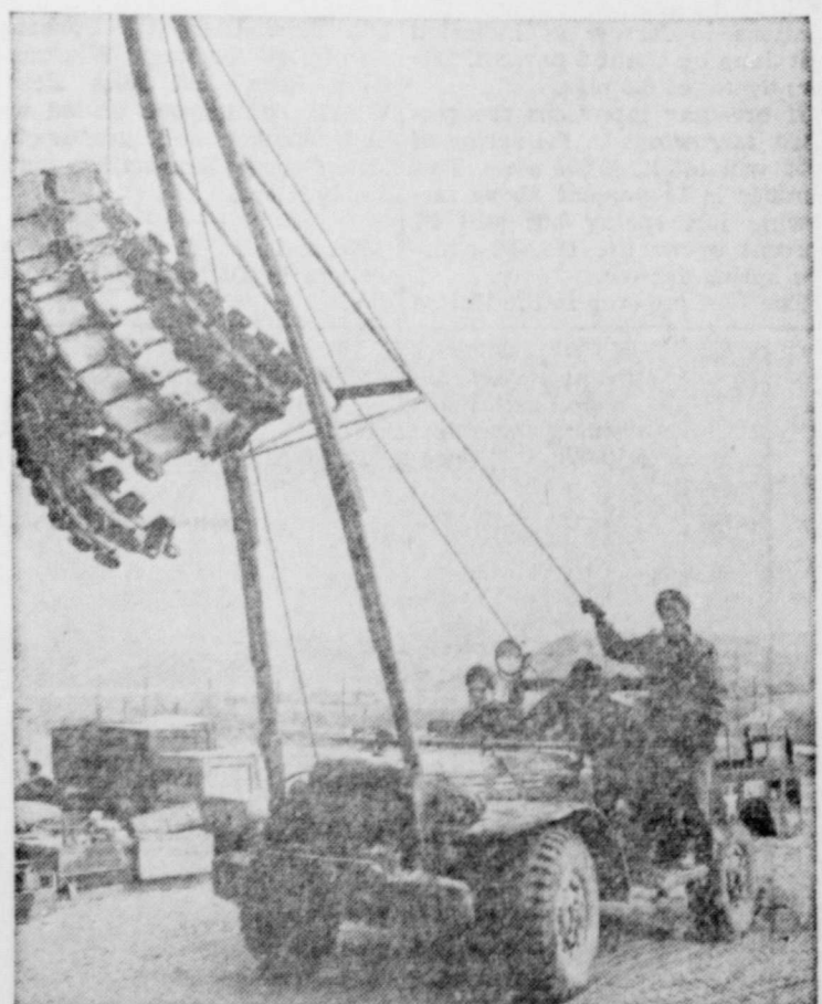
"TWO-MASTED" ARMY TRUCK sails into Korean scrap piles to salvage valuable material which can be rebuilt and put to use. Above, Army Ordnance men truck broken tank treads to repair shop.
