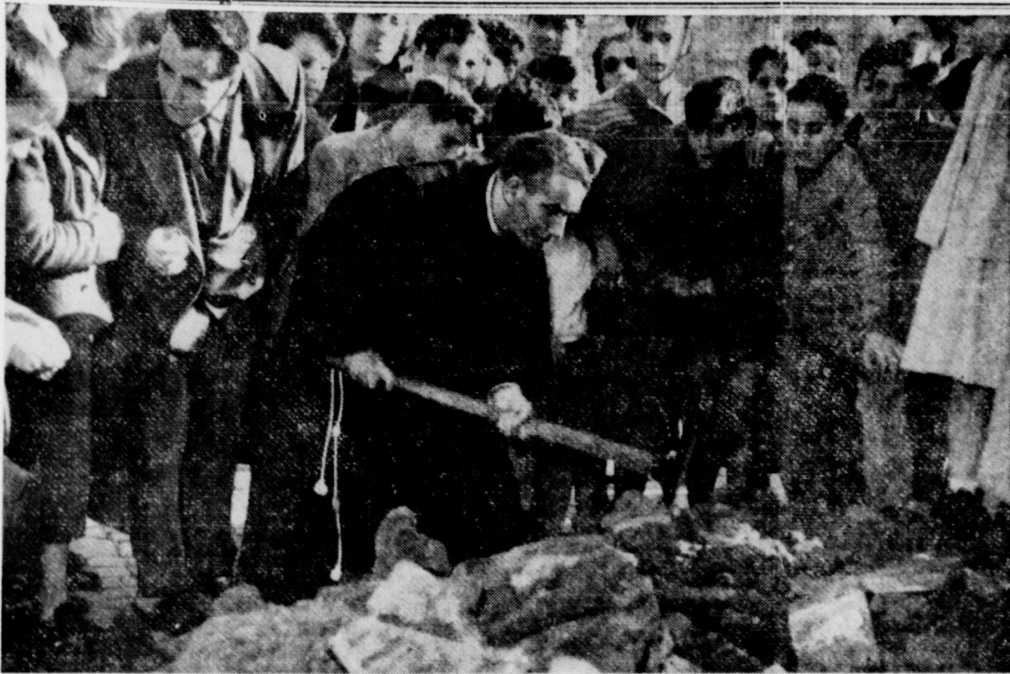
THE UNEXPECTED —A friar in Rome is using a pick to search for evidence of ancient Roman tombs in the debris of the collapsed floor of the Church of St. Chirico and Giulitta. The floor, weakened by water seepage, broke through and led to the discovery of old sarcophagi around the foundations of the church. Six persons were injured in the accident.
