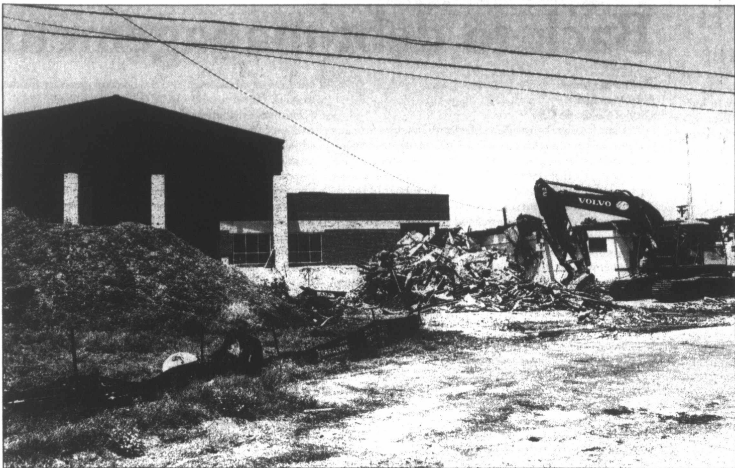
OUT WITH THE OLD, IN WITH THE NEW – Tear down of the old Loraine ISD school buildings began last week, which means completion of construction of the new buildings is nearing.
