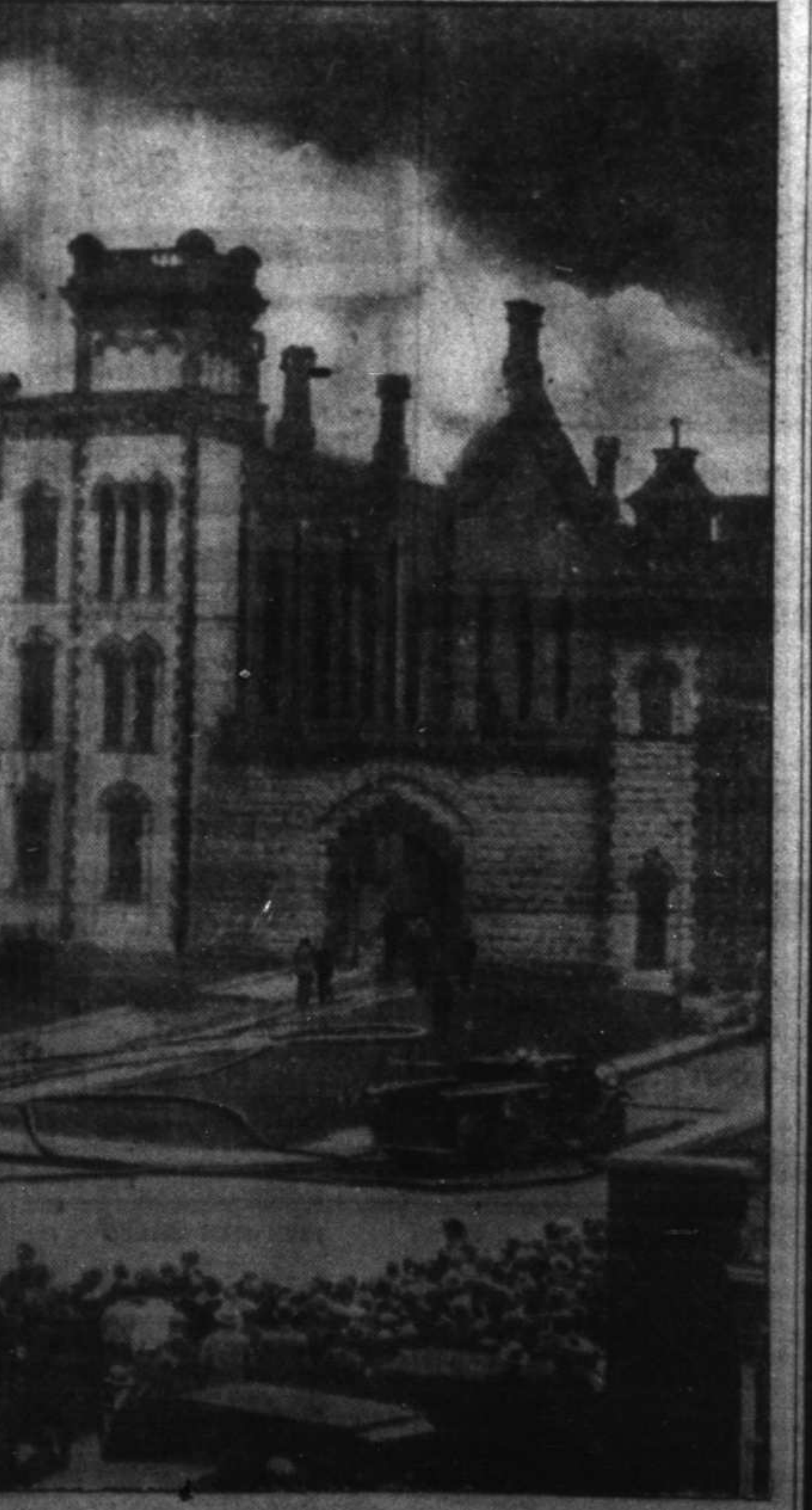
Here is another view of the exterior of the Ohio State Penitentiary at Columbus showing flames and smoke. Firemen attempted to cope with the roaring inferno in the cell block. Troops were necessary to protect firemen from convicts who resisted their efforts to put out the flames.
