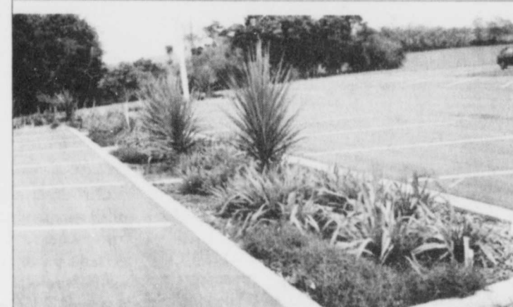
INNOVATIVE RAIN GARDENS are often a practical solution to street storm runoff for many cities. Photo courtesy of Urban Eco Construction in Atlanta, Georgia.
