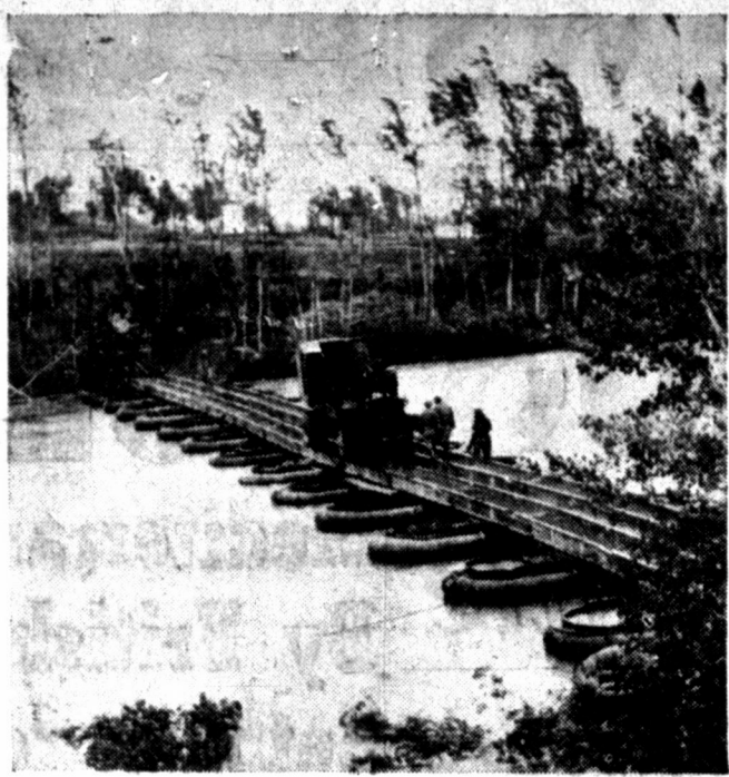
Completed, this heavy pontoon bridge became the main span for Rome-bound Fifth Army troops on the central sector of the Volturno river front. A crane is being taken across to prepare a tank landing space on the opposite shore. In background pictures of this U. S. Army bridge-building operation, Sgt. Anna was pool photographer Bert Brandt shuttled around the Volturno in a rubber boat, right.
