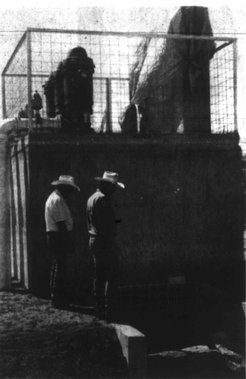
PROJECT MANAGER Glenn Hemphill and City Water Superintendent Kenneth Rich inspect the new pump station north of Champion Lake. The city's three new pump stations are now on Champion water lines and the entire water system is expected to be completed this summer.
