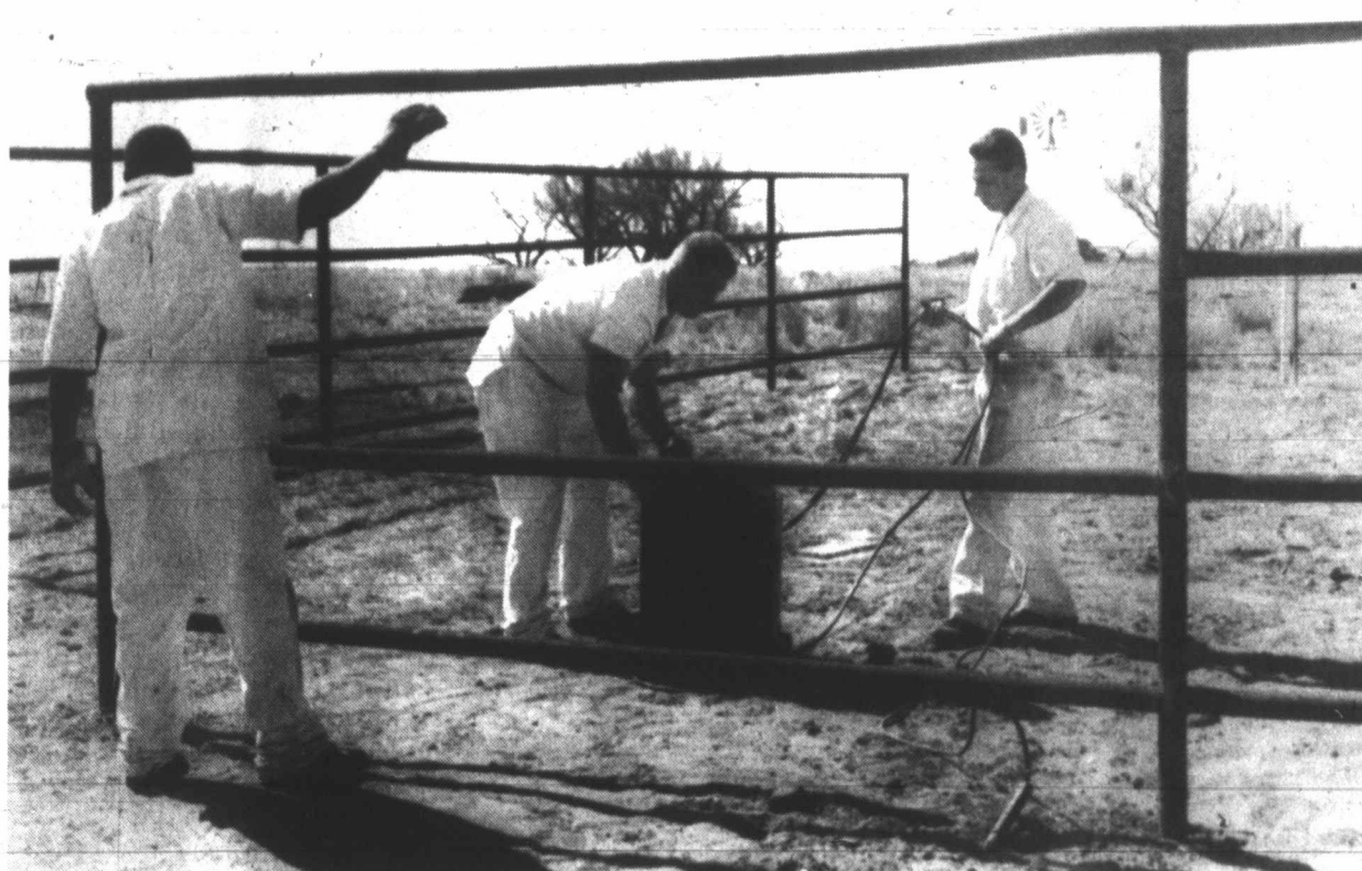
WALLACE UNIT INMATE WORK CREWS construct a corral for the Texas Longhorns at the Lake Colorado City State Park. The holding pen was made from 2-3/8 inch tubing pipe from an old oil pipe. The pen will be used when one of the longhorns has to be seen by the veterinarian and when they need to be loaded for a one-month trip to the Fandangle in Albandy this June.
