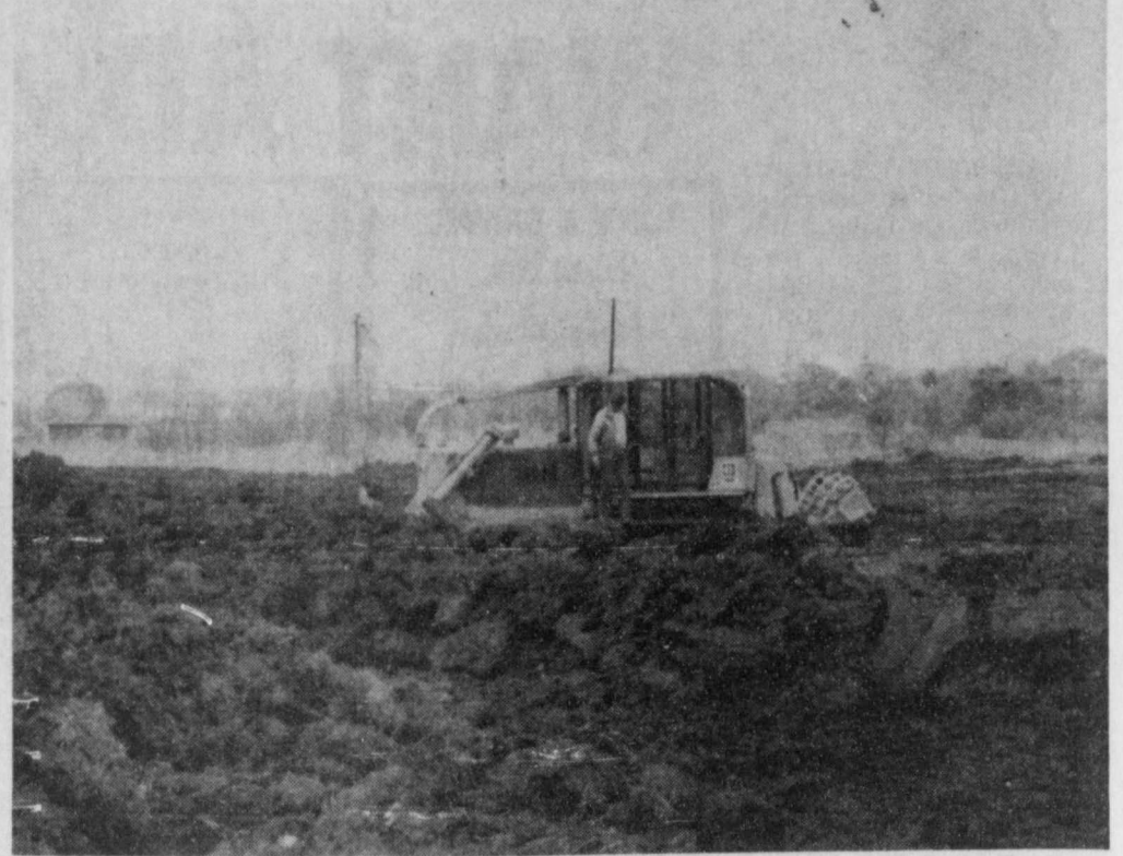
SEWFA PLANT begin'ing. It may not look like much but a lot of dirt
