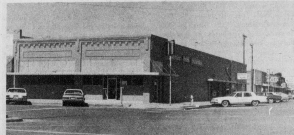
THOMPSON PHARMACY completed remodeling on the 20th of May. Walter Davis Construction laid the bricks and Wiley Griggs painted the front and the rest of the block west of Thompson's Pharmacy.
