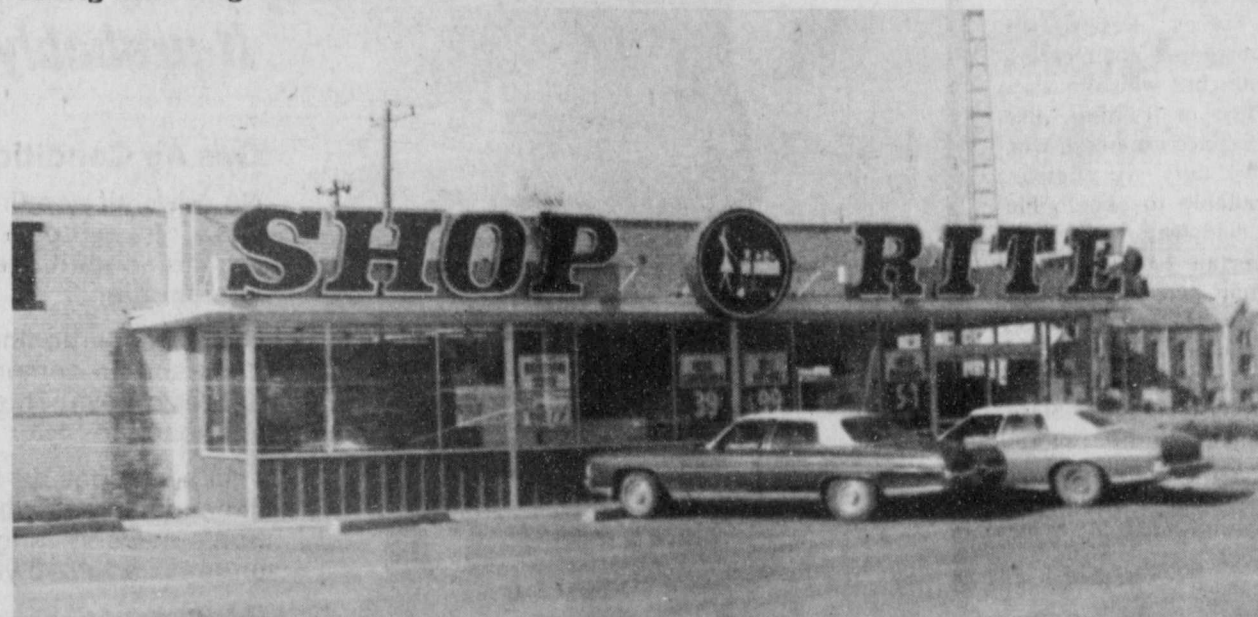
BOTH THE DRIVE and the expansion to the front of Shop Rite was completed by the last of April. Plainview Plate Glass and Mirror Company added the expansion to the front and Fred Lipham laid the new drive surface.
