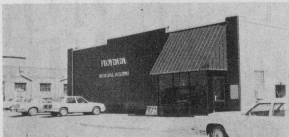
FLOYDADA CITY HALL received their new glass front the last part of April. Plainview Plate Glass and Mirror Company added to the building to help with heating and cooling the office and for customer convenience.
