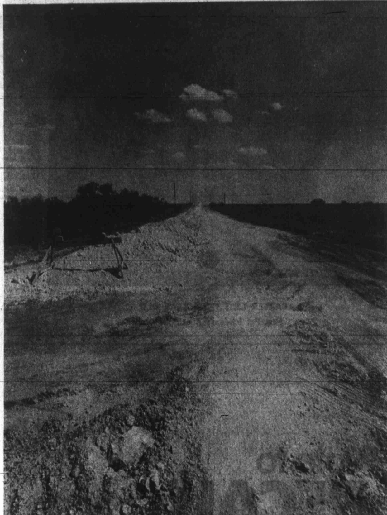
FUTURE OF THIS ROAD IS CERTAIN ... asphalt is scheduled to be poured this week
