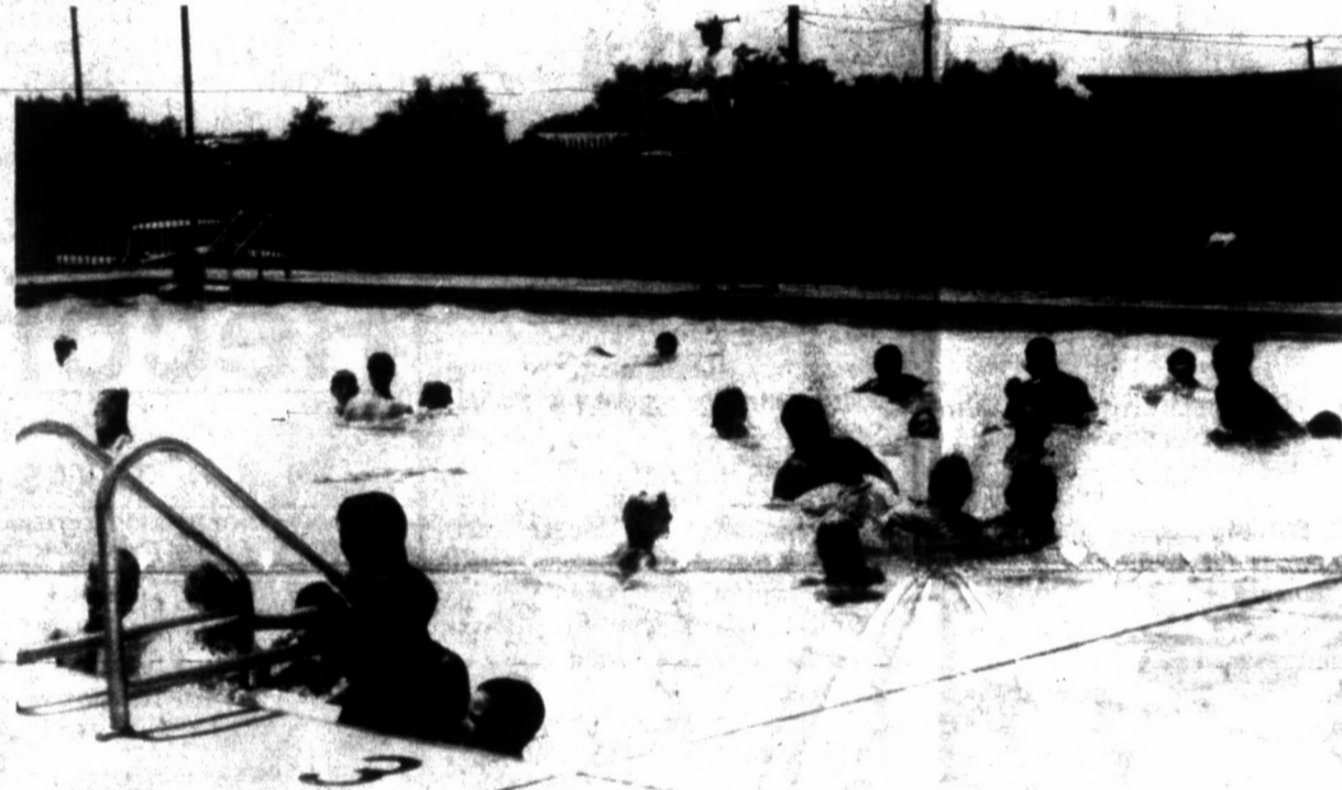
IT'S READY: The repairs to the Colorado City Swimming Pool have been completed and the water added for the summer season. A group of Mitchell County youth are shown as they cooled off from the hot afternoons.
