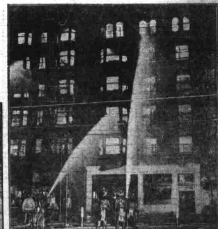
Associated Press Photo Eleven persons were known to have died, 12 others were missing and about 30 others received burns in a fire which destroyed an apartment building in downtown Cleveland. Many of the 200 residents of the building, in night attire, figured in dramatic escapes via ladders and firemen's nets.
