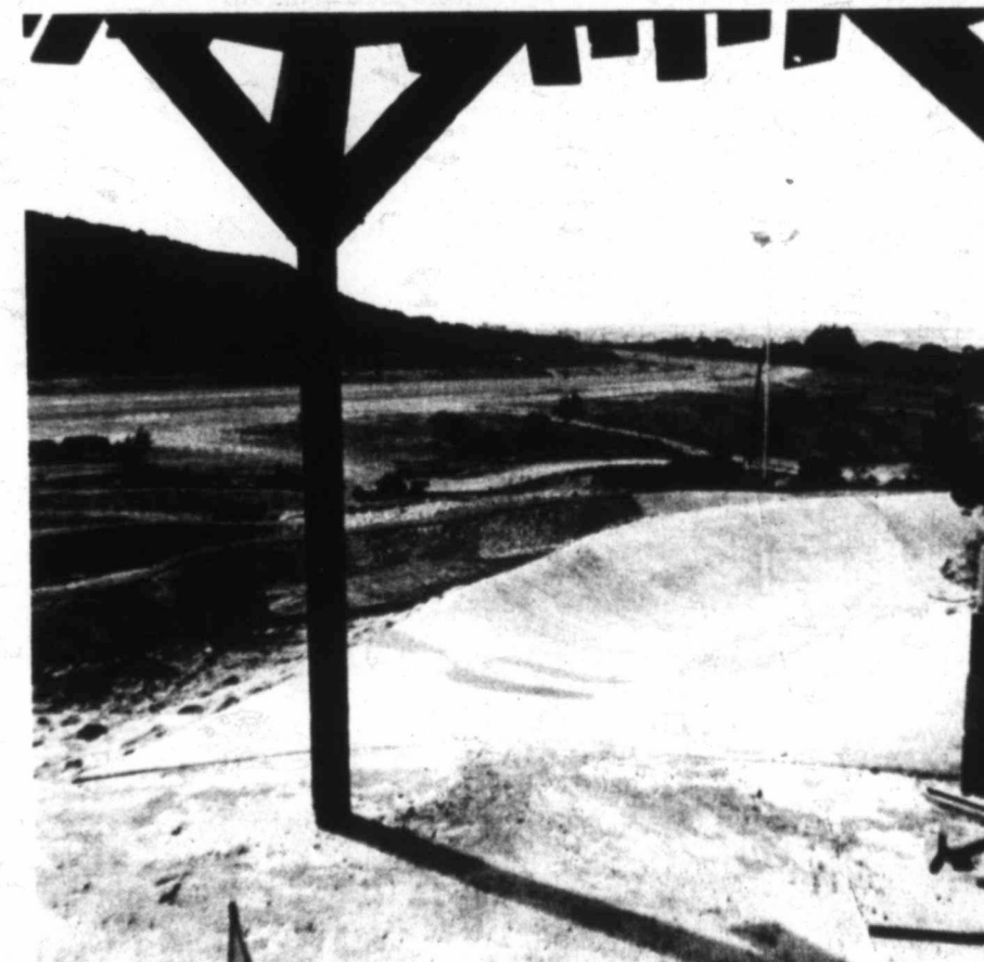
SKATEBOARDERS' DELIGHT — The concrete has been poured at the top of the highest run in this picture taken May 1. The wire in the middle of the photo was used to form and anchor the concrete to the ground. Concrete at the park covers 22,000 square feet at an average thickness of five inches. Lights are up by now, erected by Gilliland Electric Co. of Big Spring.
