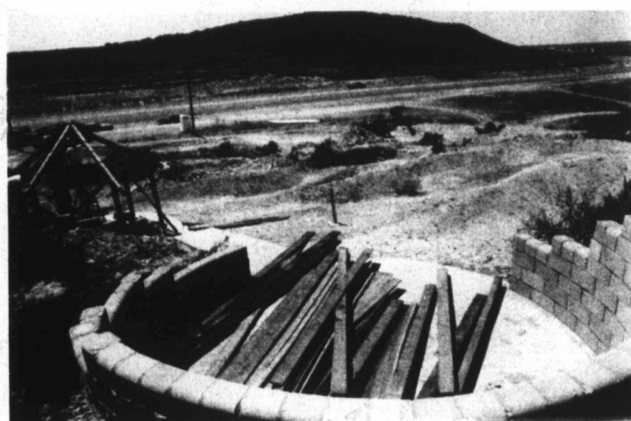
FROM THE TOP — Taken Apr. 14, this picture, taken from the top hut of the park, shows Randy Johnson and his men working on the carpentry of the lower hut to the left. The brickwork of the huts was done by John Fitts. Excavation by Marquez is still going on at this time, and the men are working around a high-pressure gas line that was not shown on any surveys of the land.
