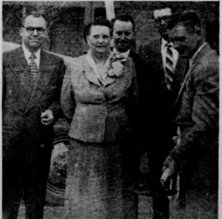
GROUND BREAKING ceremonies January 19 officially started construction of Stanton's dial telephone unit. Left to right: E. S. Ridge, traffic manager, Mamie McDurmon, chief operator, Clifford Fisher, local manager, Bill Yeatts, district manager, and Mayor Woodford Sale, turning first spadeful of dirt.
