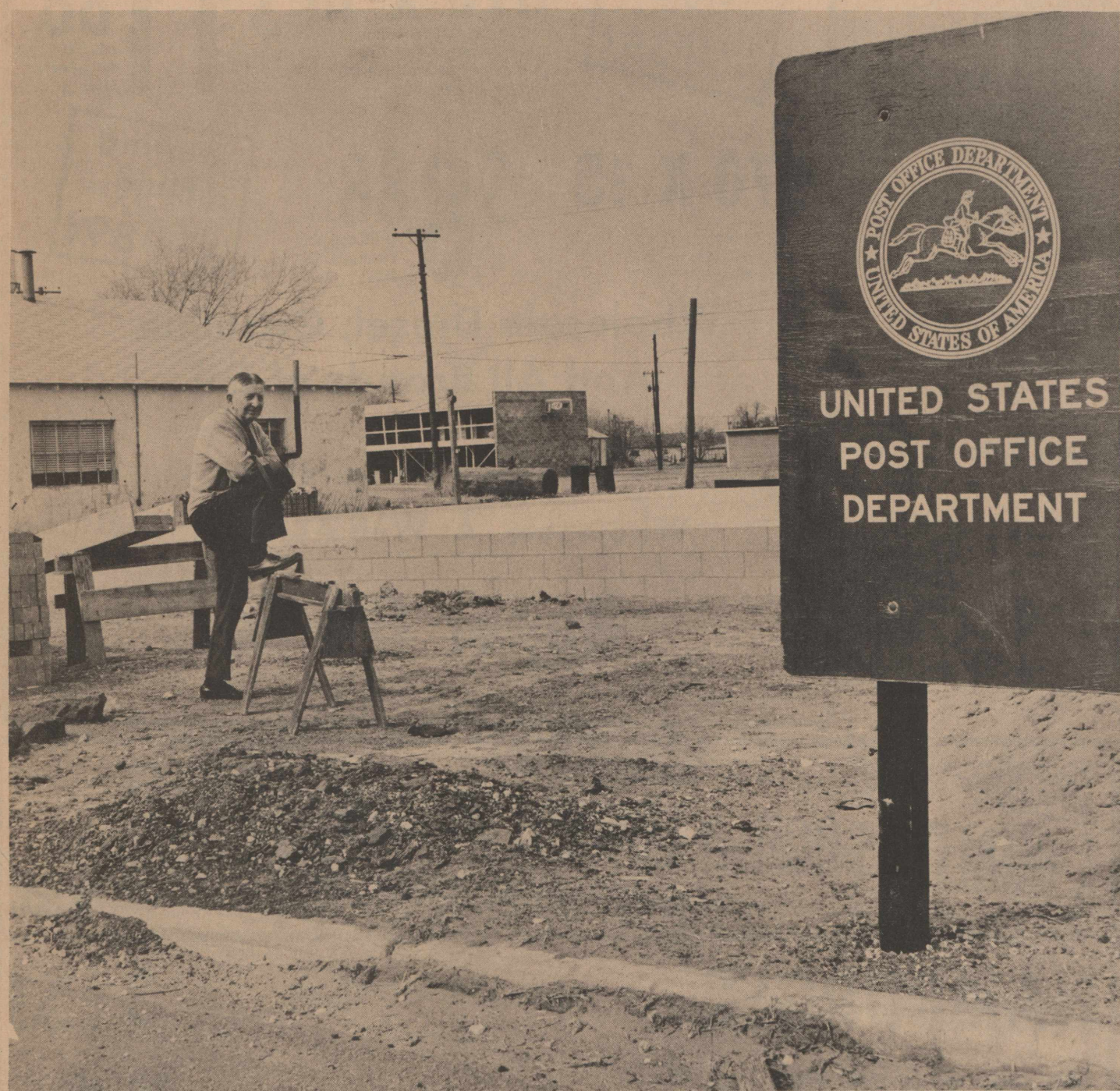
JUST A' WAITIN' ON HIS BUILDING----I.B. (Doc) HOLT, Olton postmaster, surveys the scene as he looks over construction at Olton's new post office. Floor of the new build-
