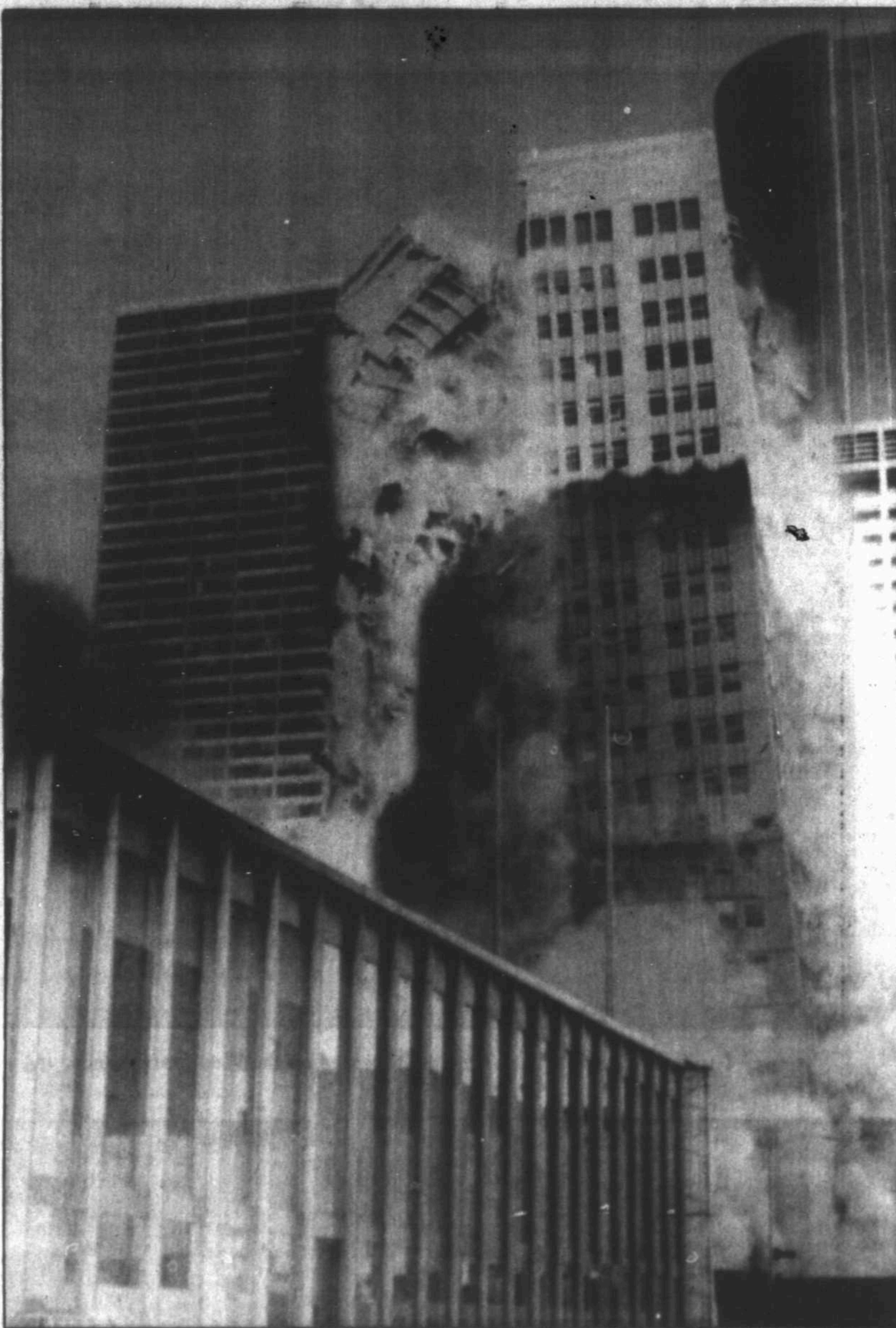
The 22-story C&I Building in downtown Houston falls Sunday as 600 pounds of explosives detonated. After the rubble is cleared, the area will be used as a parking lot.
