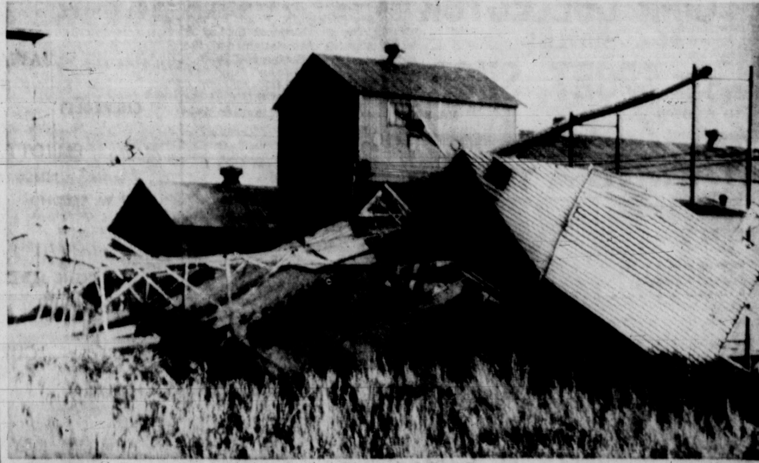
Storm Flattened Bur Box
