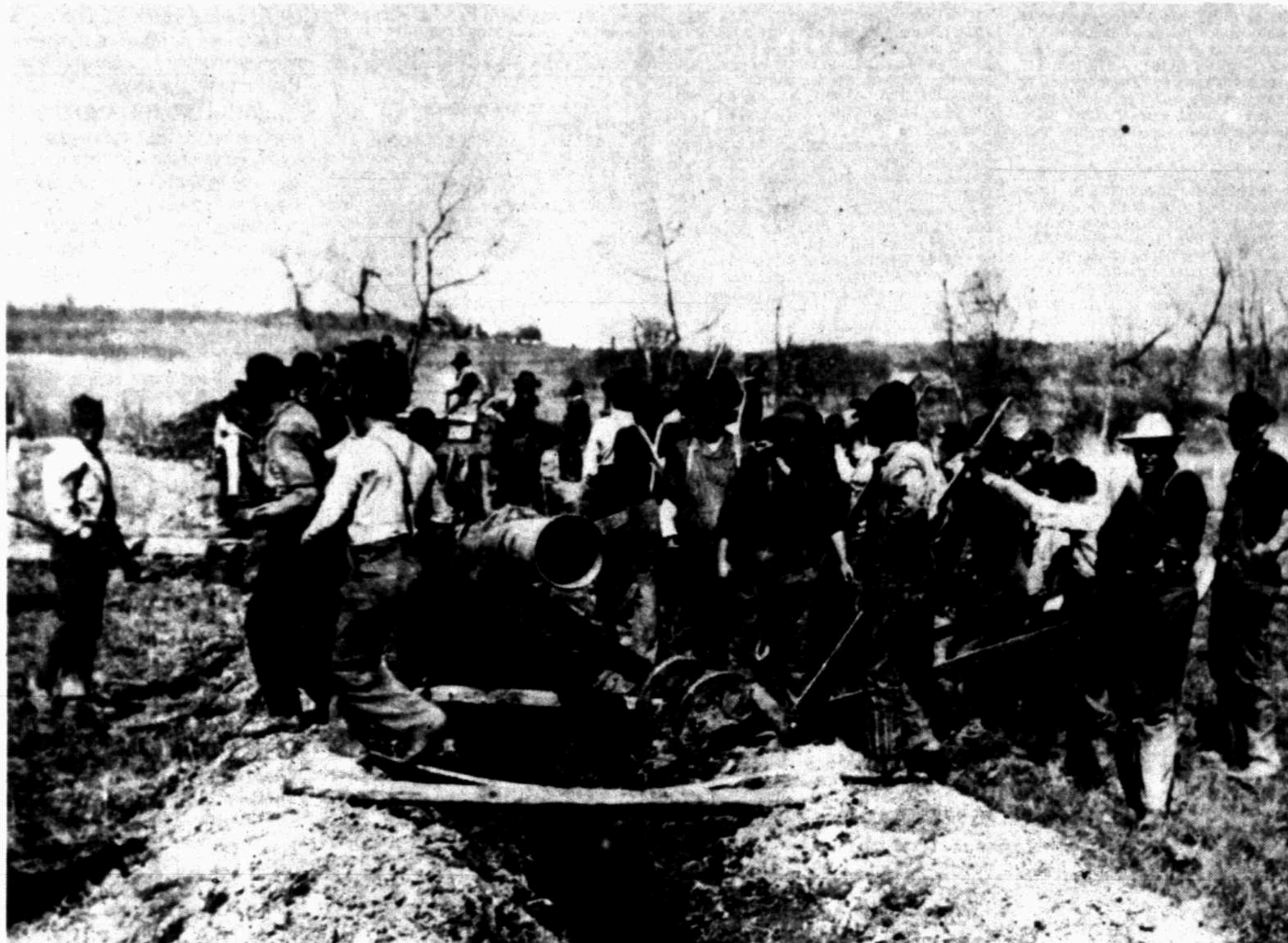
Pipeline construction gang laying pipe in West Texas. Note pipeline tongs in foreground.
