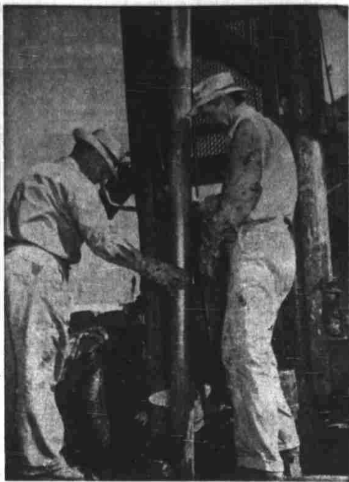
Drilling On The Town Square
