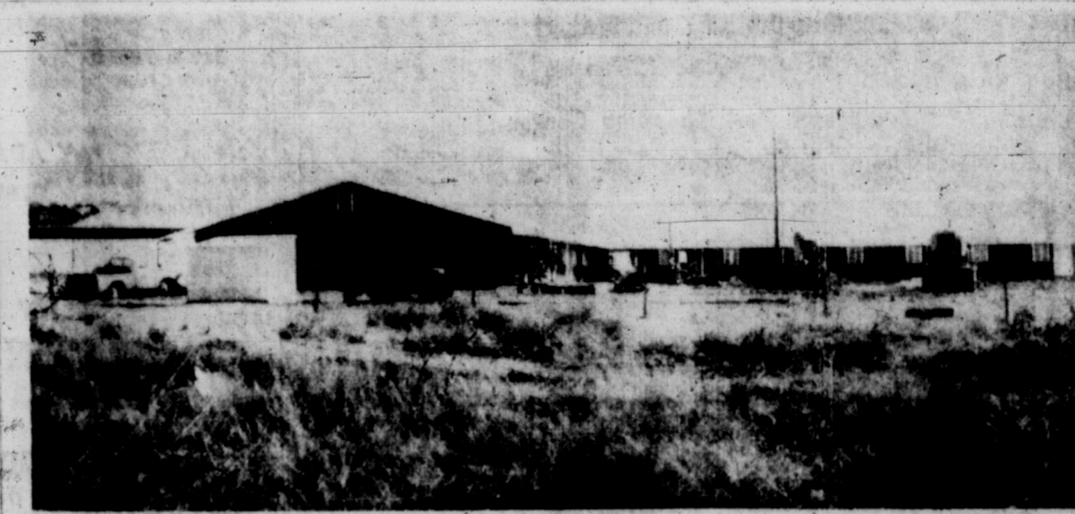
Bricking Begins Monday
