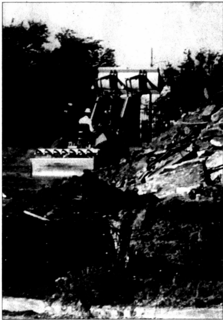
WORKERS WITH CC TANK work to clear the land on Pine Street where the new jail will be located. The project is expected to last a year.
