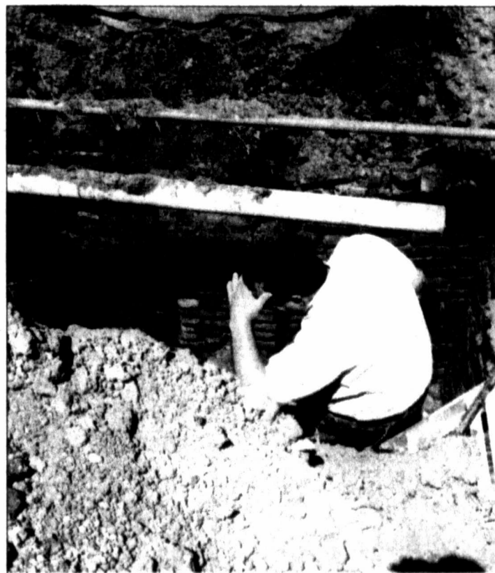
JUST UNDER FOOT — Colorado City Code Enforcement Officer David Hoover inspects an underground cistern which opened up last week, surprising the workers who were working on top of it.
