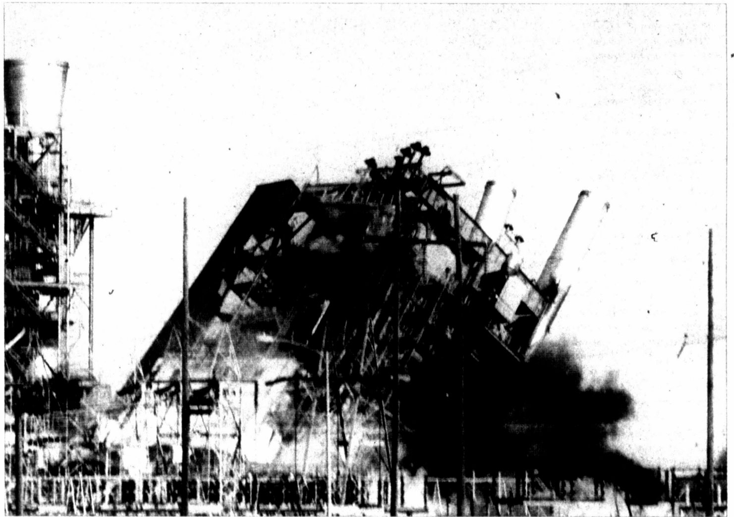
FALLING DOWN — One of the two remaining natural gas steam units at Luminant's Morgan Creek Power Plant was imploded Friday morning. The remaining steam unit is planned to be demolished as well, but a date and time has not been determined for that to take place. (Staff photo)
