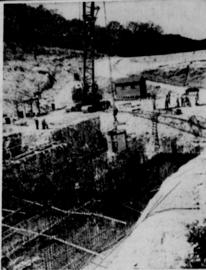
FIRST CONCRETE —Concrete is being poured on the Belton dam project (above) for the foundation of a 200-foot control tower. The tower will connect with an 800-foot conduit to handle flood waters on the Brazos River. A public ceremony is planned when concrete is first poured on the dam itself. (UPI Photo)
