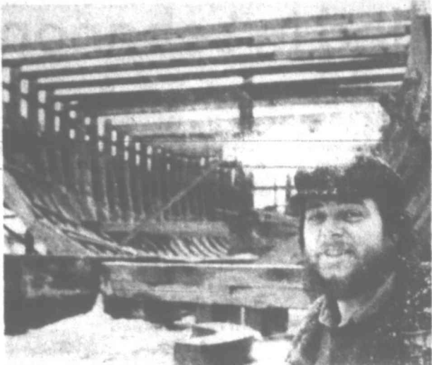
(AP WIREPHOTO) CARGO SCHOONER TAKING SHAPE — Ned Ackerman stands in front of the 97-foot schooner he's building in Thomaston, Maine. The two-masted vessel will have a 23-foot-beam and will be used as a cargo carrier in Atlantic waters. Ackerman hopes to have the schooner completed late this year.
