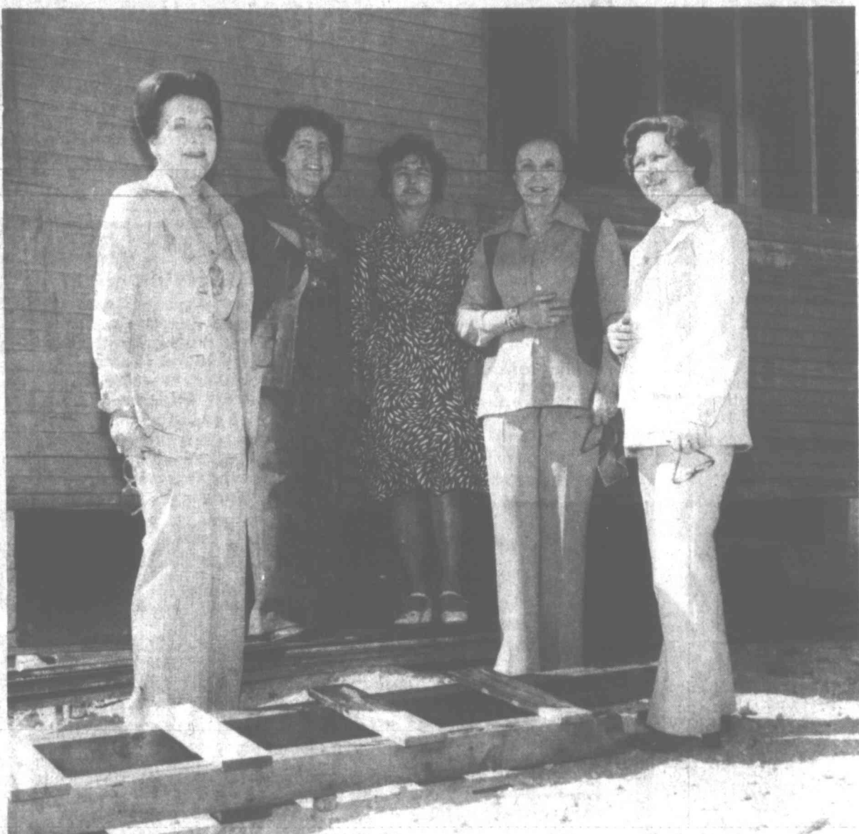
IT DOESN'T LOOK like much now, but people are beginning to put some effort into turning this building into the Northside Day Care Center. Here, members of the Permian Basin Medical
