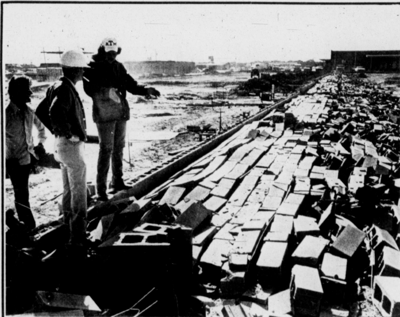
HBF Builders' Travis Melton, left, Troy Melton, center, and Butch Keith survey the damage at 3300 N. Midkiff Ave. (Photo by Bruce Partain)
