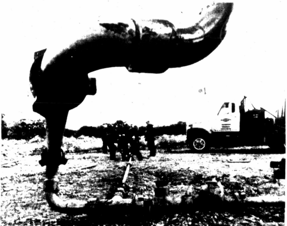
The most hazardous conditions prevail in the field and employees tackle each job with precaution.
