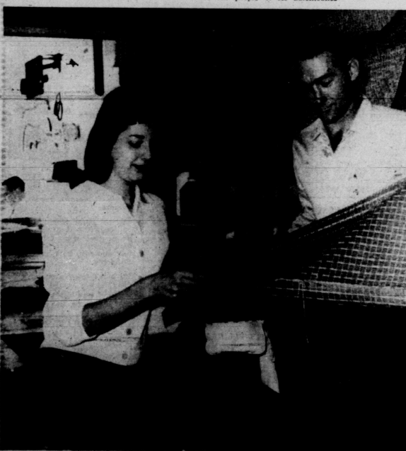
WINDSHIELD, GLASS AND MIRROR SHOP —Bill Lawton, manager of the Windshield Glass and Mirror Shop located at 1701 Twenty-fifth Street, shows Ora Beth Henderson, 3001 Thirty-ninth Street, some of the new seat cover fabrics that have just arrived at the shop. The firm features fast, complete service on all automobile glasswork, custom seat covers, headlining, and carpet.
