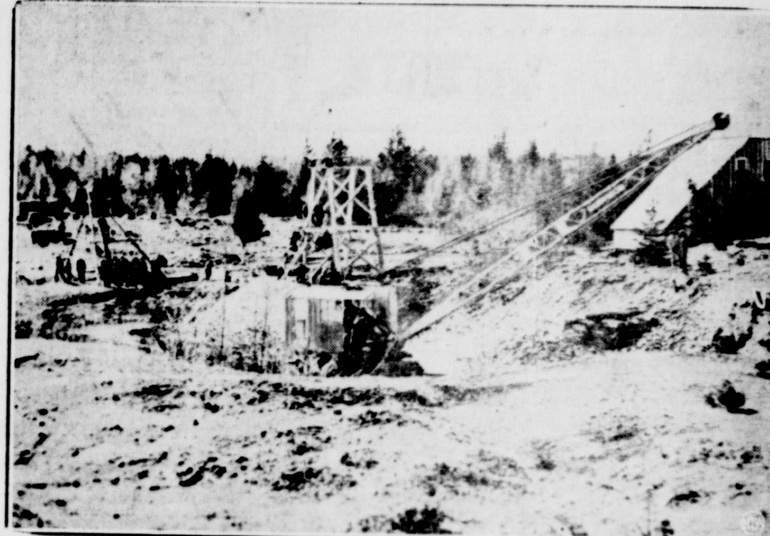
Three hundred men worked feverishly at Moose River, Nova Scotia, to reach three men trapped for more than a week 140 feet underground by a cave-in in a gold mine they were inspecting. Pictured at the scene of the disaster is the big steam shovel used to speed up excavation.
