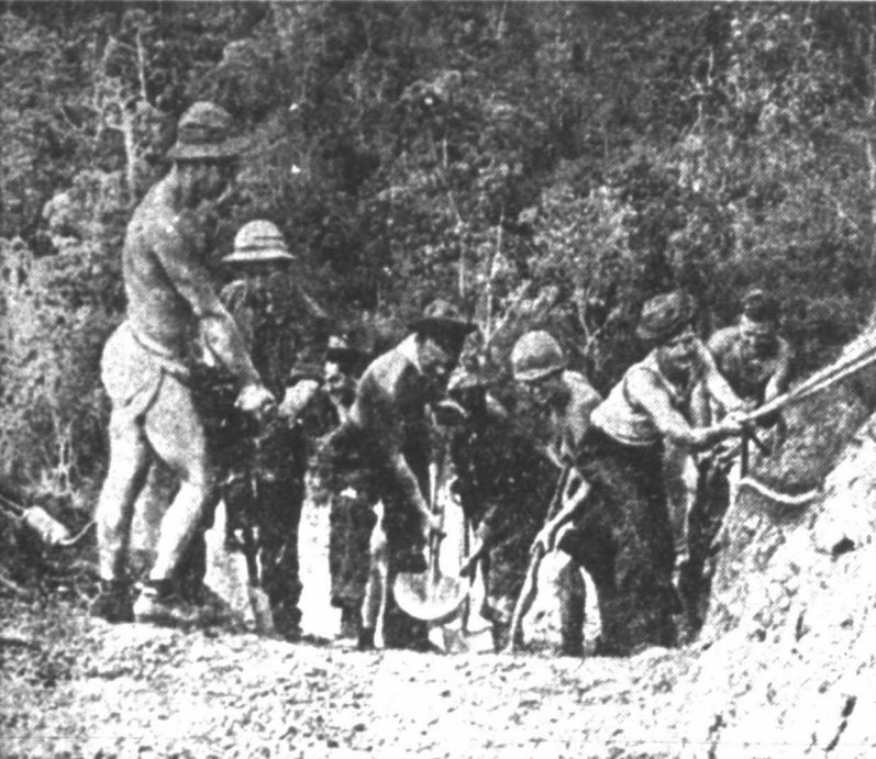
Building "Pee" roads in New Guinea is all part of the day's work for American army engineers. This particular road under construction near Port Moresby, main Allied base in New Guinea, is so steep that the men must hold on to ropes to keep from falling backward. The grade drops about 65 degrees behind them.
