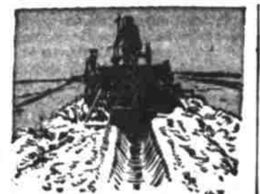
Ditch-digger, machine at work.
