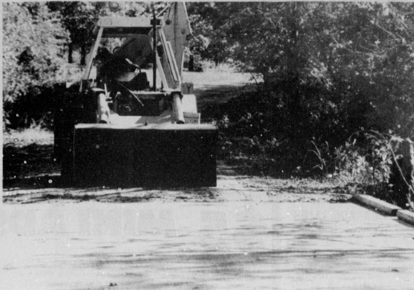
NEW BRIDGE —The 80 foot bridge on the old Johntown highway has a new concrete surface and is ready for traffic. The bridge has been closed for a week allowing
