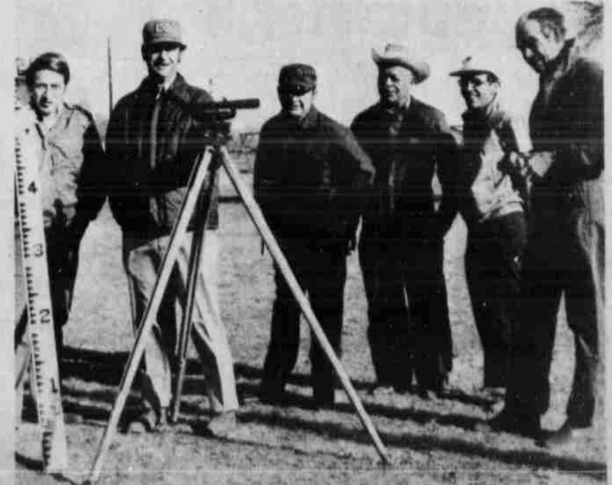
A NEW BASKETBALL COURT will soon be in place in Dunbar Park, located in the northeast section of Littlefield. Some of the men involved in the project are shown staking out the court Saturday. Forms were laid Wednesday and cement will be poured Friday. Goal posts will be erected later next week. Work crew members are, left to right, Byron Ford, project chairman, David Hamblin, Harold Heller, Bert Wasson, Lloyd Lust and Bryson Kisner. (Staff Photo)
