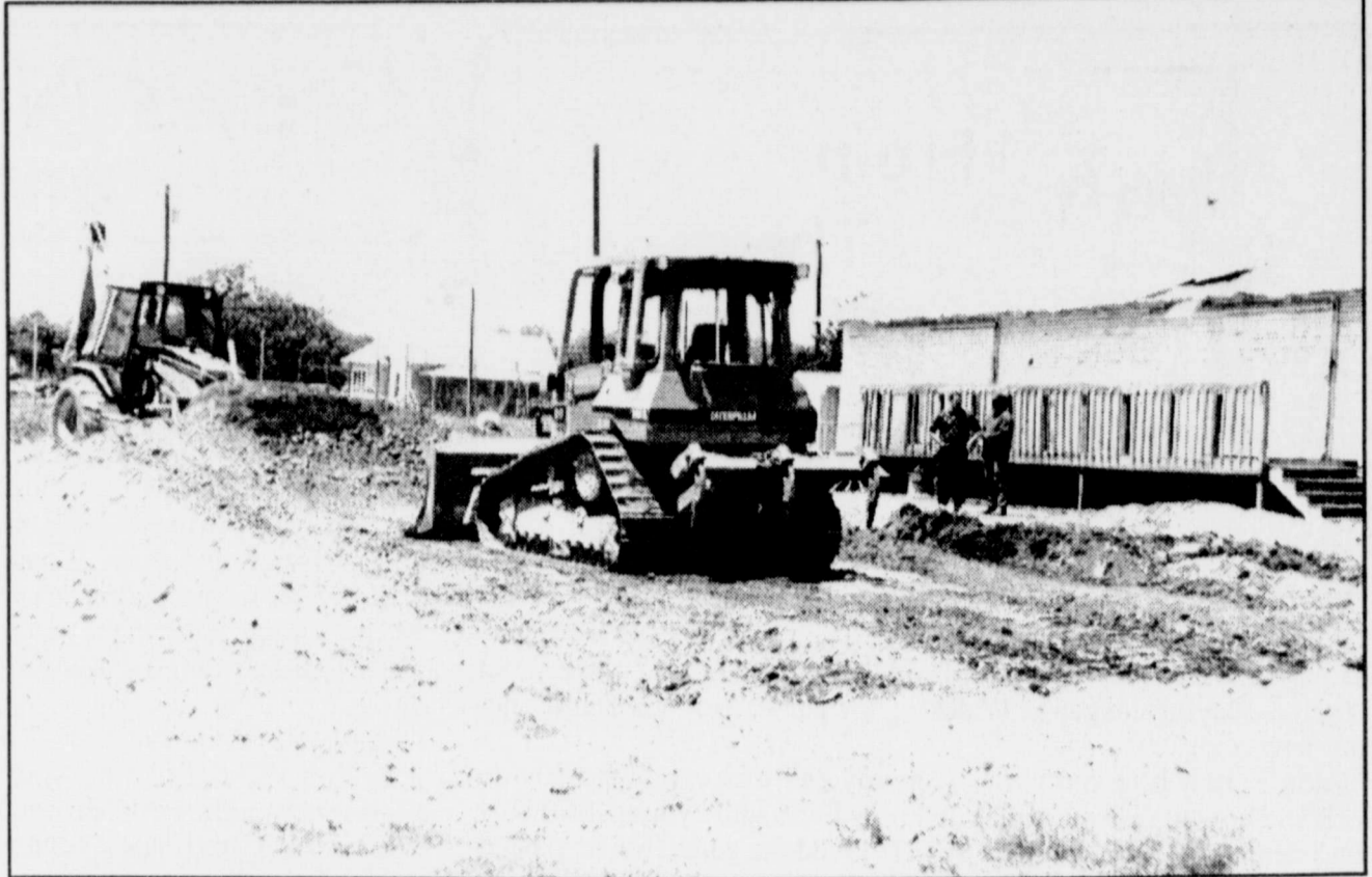
SAND VOLLEYBALL COURTS are being constructed near the First United Methodist Church as dozer work donated by Bishops & Sons was underway last week.
