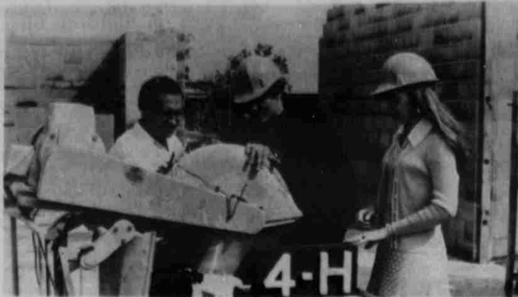
CENTER TAKING SHAPE — Eddie Perkins of Cleburne (center) and Jamie Hemphill of Coleman, chairman and vice-chairman, respectively, of the Texas 4-H Council, inspect a masonry saw with Job Supt. Ed Miller of the Herman Bennett Company while on a special inspection tour of the $1.375 million Texas 4-H Center at Lake Brownwood. The 200-capacity facility is being constructed under the leadership of the Texas 4-H Foundation and is expected to be completed by early spring 1975.
