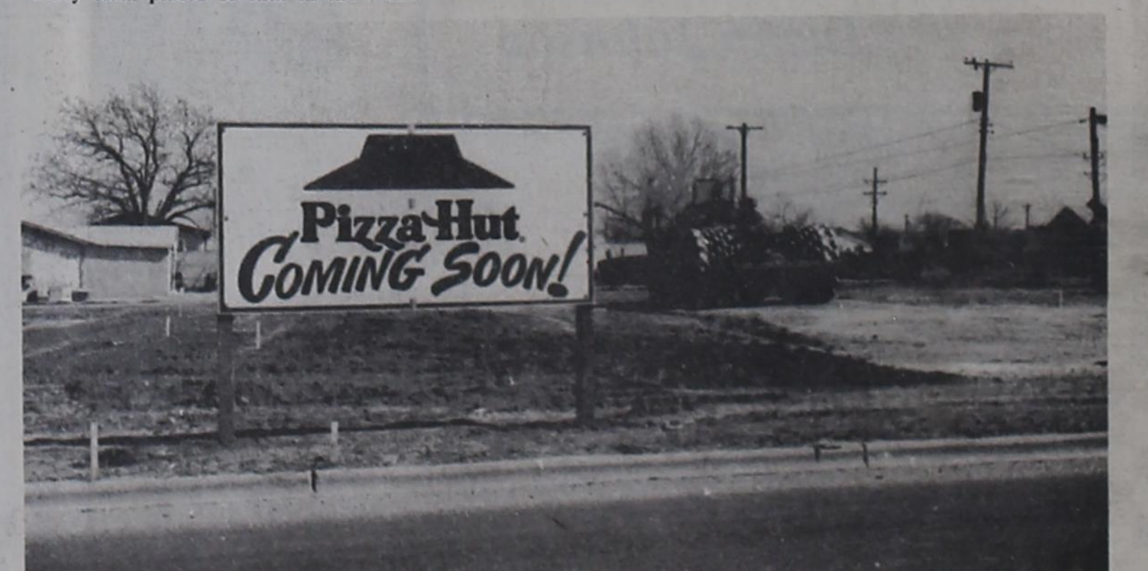
BUILDING PERMITS were issued last week to Pizza Management Inc. of San Antonio for the construction of a Pizza Hut in Post. The site is being prepared at the 300 block of South Broadway. Pizza Management Inc. district supervisor Larry Hopp of Lubbock announced that the facility should be open in April.
