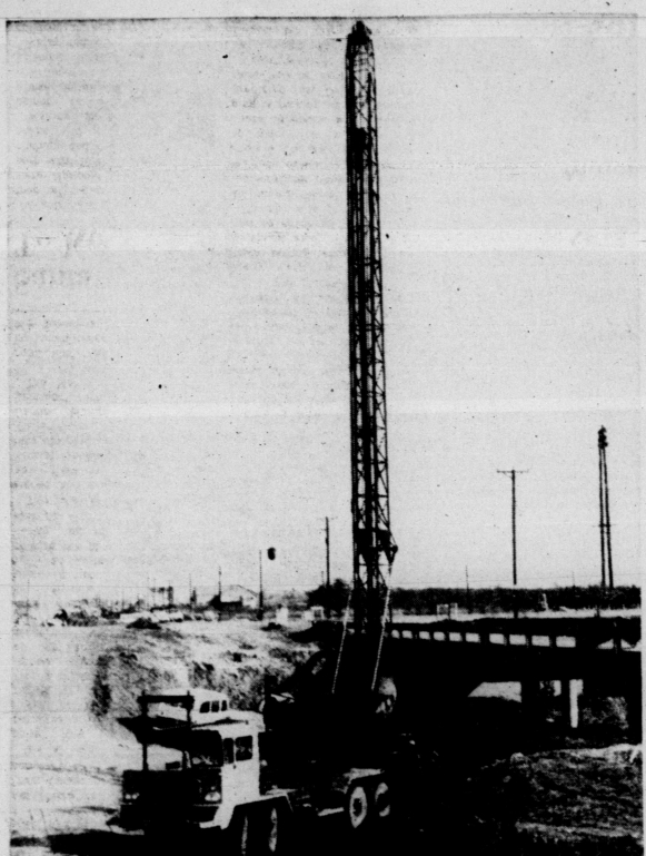
DIGGING IN DEEP CREEK —Widening the bridge over Deep Creek on Thirty-Seventh Street near Avenue M called for drilling holes, some 25 feet deep for supports. A giant bit 2 feet wide bored sometimes for half a day on one hole, casing it for the concrete crews. In the background above is the covered Avenue M traffic light that has temporarily been replaced by a stop sign. The highway department has suggested that traffic detour by way of Thirtieth Street as much as possible, although the road has been closed only to through traffic. Construction of another bridge can be seen in the background.
