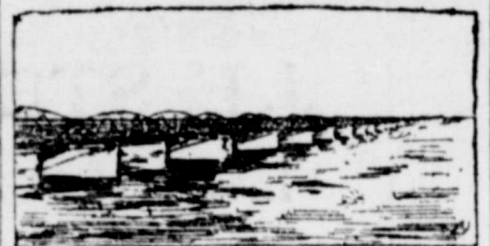
BRIDGE OVER GALVESTON BAY.
