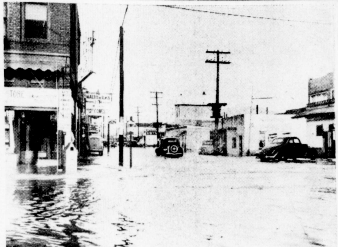
Flooded street scenes in Picher, Oklahoma, at 8 o'clock Saturday morning. Picture shows flooded Picher, which was one of several towns isolated by high waters. Highway and train service both were disrupted. Heavy rains sent creeks and rivers out of banks inundating thousands of acres of land. (NEA Photo).
