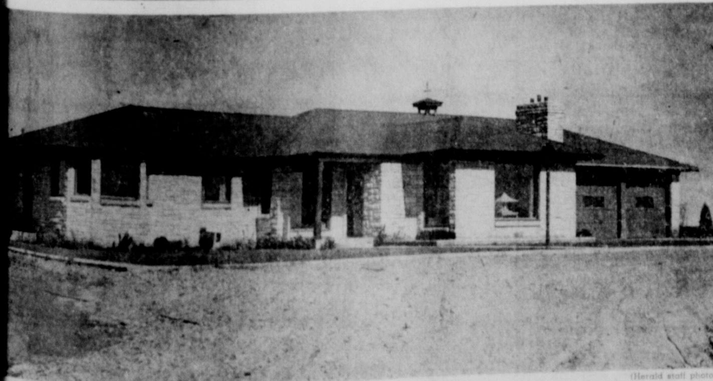
GEORGE HOME Every Modern Facility for Comfortable Living
