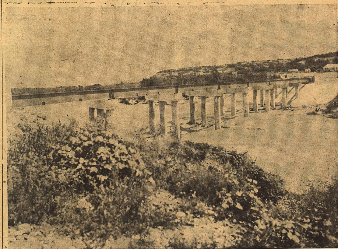
This 320 foot bridge over the Devil's River is part of the Sonora-Eldorado highway project to be completed in mid August.
