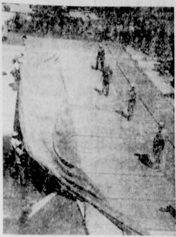
ROLLING OUT THE CARPET —Sixty feet below the surface of the ground in downtown Houston, workers stretch out a Butyl rubber carpet on which the 44-story Humble Oil & Refining Company building will stand when completed in 1962. The Butyl membrane will act as a water barrier for the foundation of the building. This is a unique application of the durable, flexible synthetic which is produced at Humble's Baytown Refinery and is widely used in everything from hot water bottles to conveyor belts, tubing, tires, wading pools, protective clothing for missile launching crews, and car accessories.
