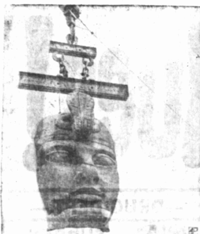
MILLENNIAL MOVE — The great stone head of Ramses II, in situ for 3,000 years, is lifted after being cut from Abu Simbel temple to make way for the Aswan Dam.
