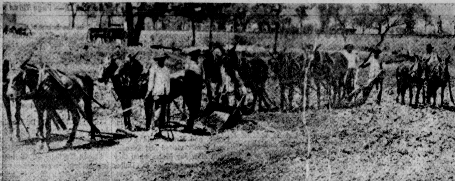
THIS IS A STOCK TANK — When they built stock tanks back in 1905, they did it the hard way, with some strong men, sturdy mules, and "slips." Clinton Busby, 813 Fig, brought in this early day shot. Among peo-
