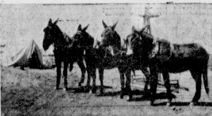
HIGHWAY BUILDING, 1925 STYLE — In early road-building days in West Texas, highway building would have been impossible without the help of such mules as Elick, Kate, Charlie and Bob (left-right), the four mules pictured above. The picture, made in 1925, was submitted by Mrs. J.U. Dawson, Route 5.
