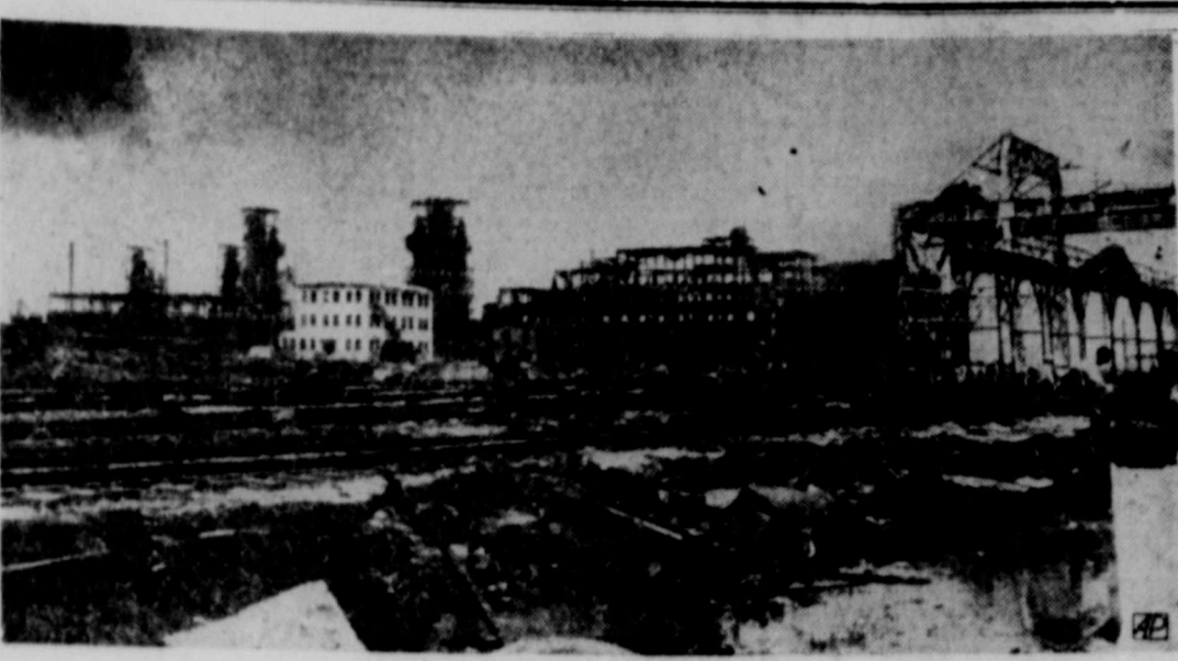
DESOLATION AFTER BLASTS—This desolation, reminiscent of war scenes, is the remnant of the Monsanto Chemical plant at Texas City on April 21, five days after explosions and fires which ravaged much of the Texas coastal community. Company officials have announced that the plant will be rebuilt on the same site. (AP Wirephoto)
