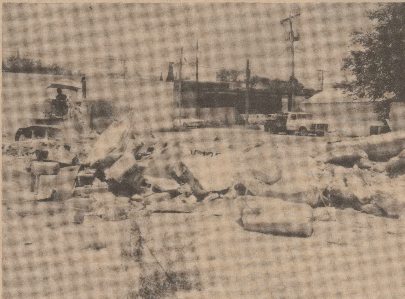
MAKING WAY FOR PROGRESS —The old Perner building which housed North Grocery for so many years and more recently Western Auto, was torn down this week to make way for a parking lot in downtown Ozona. Ozona
