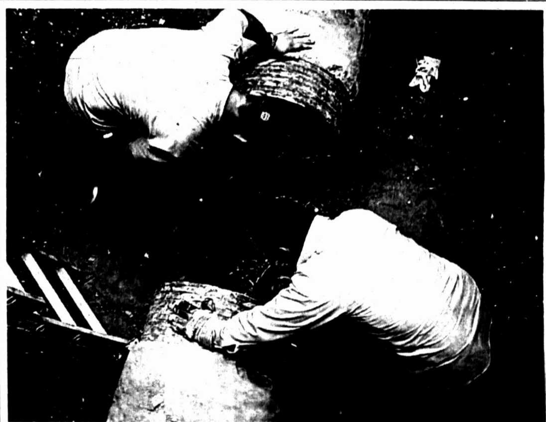
Randy Roach, top, and Albert Garza, city water department employees, inspect and prepare the cut ends of a 20-inch water main. Work crews were replacing a valve in the main — located at the intersection of Baylor and Kentucky Way — this morning, and expect water to remain shut off in the area until 5 or 6 this evening.
