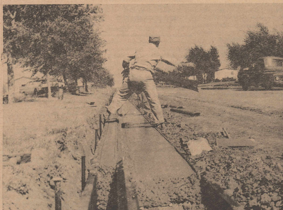
HART STREETS, 12 blocks, are now in the process of being paved. At present the crews are laying concrete for curbs and gutters, as shown above. Asphalt paving is expected to be laid in the near future. Streets under construction are Avenues F, G and E, from Broadway to First Street. (STAFF PHOTO)
