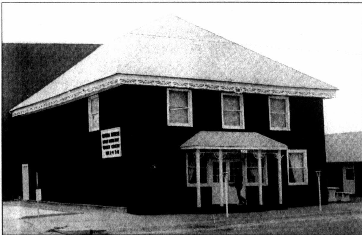
THE COLORADO CITY OPERA HOUSE is officially open again at 337 Walnut St. with the presentation this weekend and next weekend of the comedy, "Don't Drink the Water." It is the 101st theatrical production here since the 1960's.
