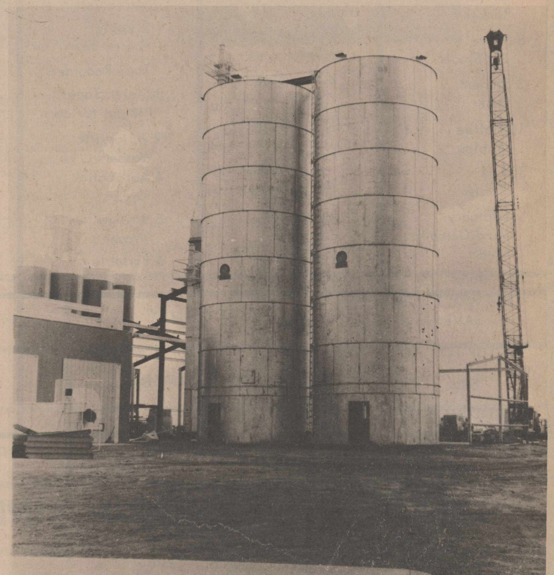
GRAIN STORAGE TANKS at the Olton Feedyards, Inc. reach toward the sky as the construction of the enterprise continues. To the left of the grain storage is shown a part of the mill. Completion date has been set for Nov. 1 and representatives of the mill said they felt that the mill would be in operation by that date. (STAFF PHOTO)
