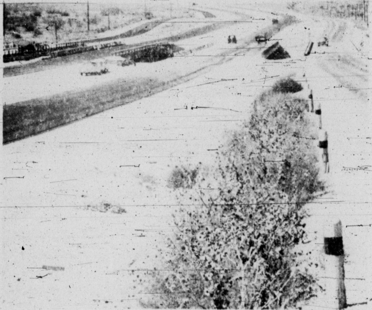
HIGHWAY PROGRESS —Paving nears completion on the stretch of U. S. Highway 80 freeway being constructed west of Colorado City to the Howard County line. The section of highway shown is approximately four miles from here where the freeway crosses Morgan Creek.
