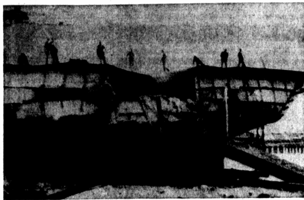
AUSTRALIAN SPAN FALLS — Section of bridge and crushed concrete pylon are viewed by rescue workers after a bridge under construction in Melbourne, Australia, collapsed today killing at least a score of workmen and injuring almost as many.
